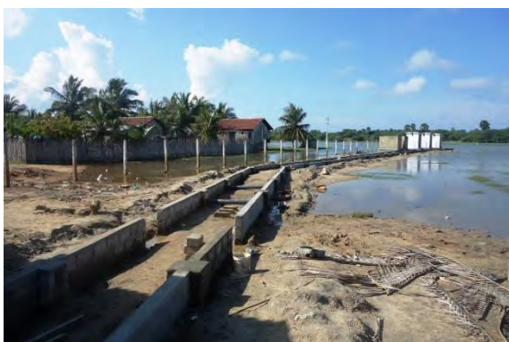
Form work completed
